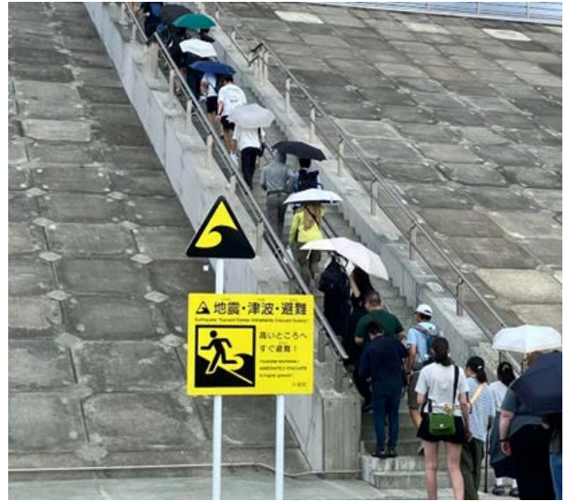
Photo: ANU and University of Tokyo students climb the 14.6-metre seawall built to protect the town of Ōtsuchi in Iwate Prefecture from tsunamis.
